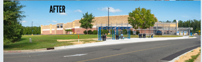
Glenn View Bus Stop Installation Project
